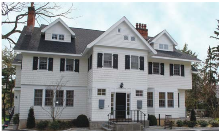
The overall look of the house was changed when the Howards took off the siding and rearranged the windows.
